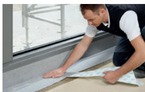
Joining window to base plate
