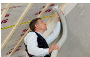
Mounting vapour control layer for injection insulation
