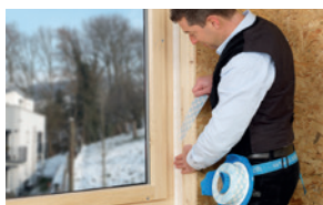
Joining window to timber wall construction
