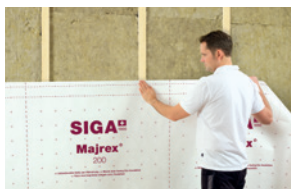
Mounting vapour control layer on timber substructures
