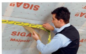
Vapour control layer overlaps
