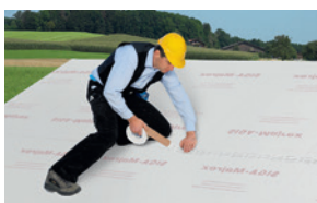
Mounting vapour control layer for above-rafter insulation
