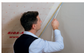
Joining vapour control layer to solid wall construction
