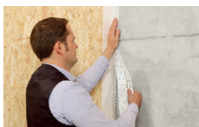
Joining timber to solid wall construction
