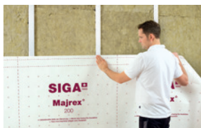
Mounting vapour control layer at internal insulation
