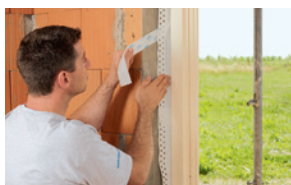
Joining window to solid wall construction
