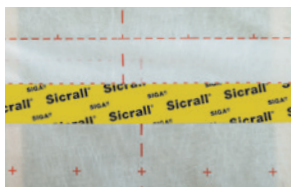
Vapour control layer overlaps
