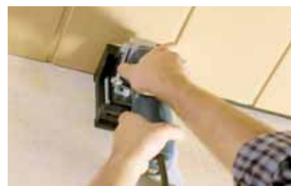
cutting of shadow joints
