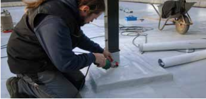
Manual welding with plastic sealing sheets.
