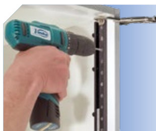
Drilling for placing shelves.
