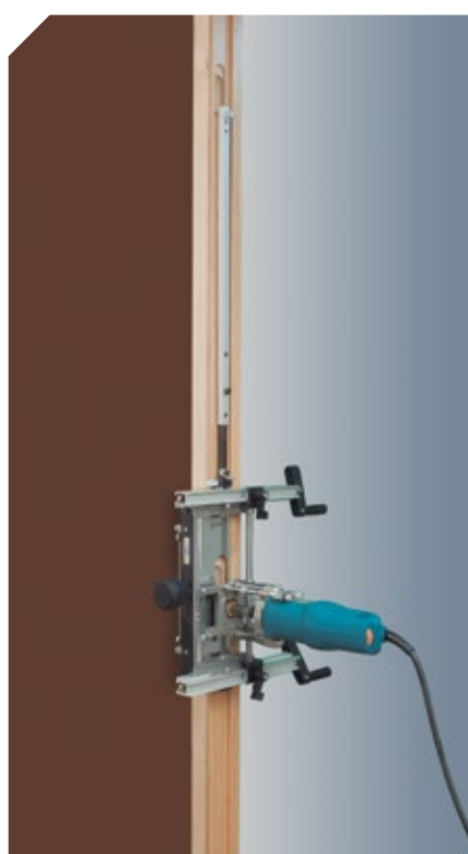
Making the second recess on the frame.
