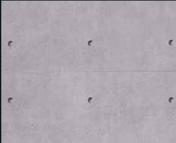
M-171 · Concrete Wall Panel Panel Cemento Encofrado
