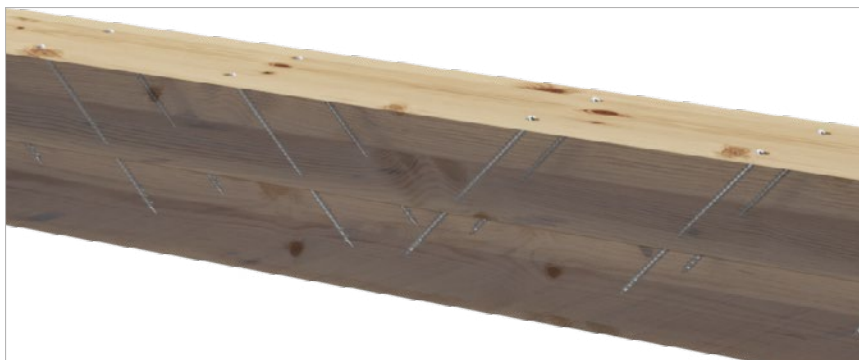
Reinforcement by coupling of beams
