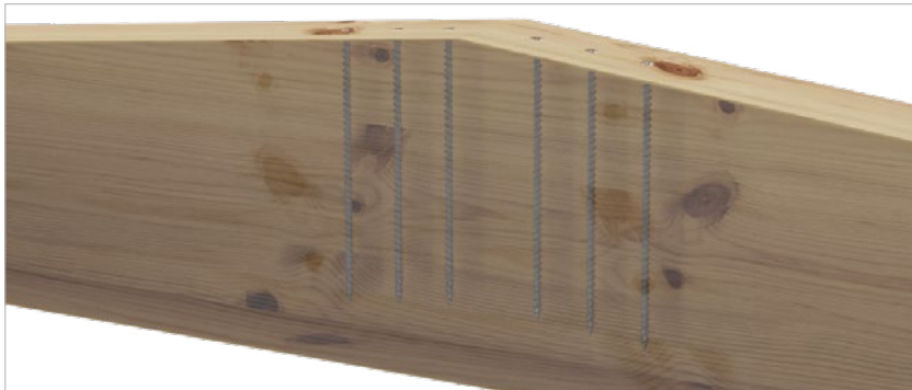
Reinforcement with screws in roof ridge area
