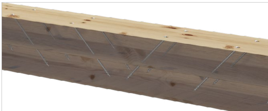
Reinforcement by coupling of beams
