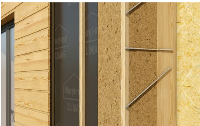
Fixing of insulation on façade
