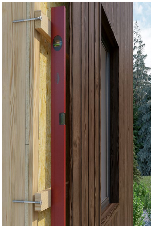
Levelling of facade substructure
