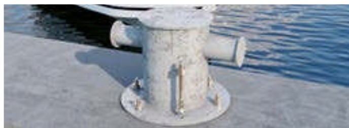
LE-A4 - Wedge anchors (Stainless steel A4)
