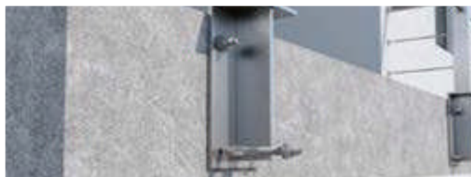
LE-DA4 - Wedge anchors (SQ Ceramic + Stainless steel A4)
